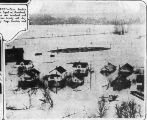
VENICE HAS NOTHING ON OREGON CITY—When the Willamette river goes on the rampage and sweeps the valley of the same name, inundating Oregon City and destroying thousands of dollars worth of property. Hundreds of homes were flooded. Photo shows outskirts of Oregon City under water.
